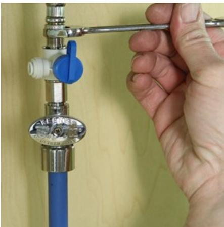
3. Be sure the blue handle on the angle stop valve is in the closed position (as pictured). Now open the sink shutoff valve and check the angle stop connections for leaks. If there are leaks repair them now. If there are no leaks connect the orange tubing to the angle stop valve. Leave the other end of this tubing unconnected for now, it will be connected later in the installation.
