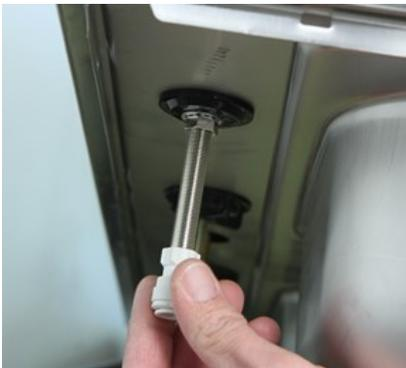
3. Now push the blue tube into the faucet connector. Leave the other end of the blue tube unconnected for now, it will be connected later in the installation.
