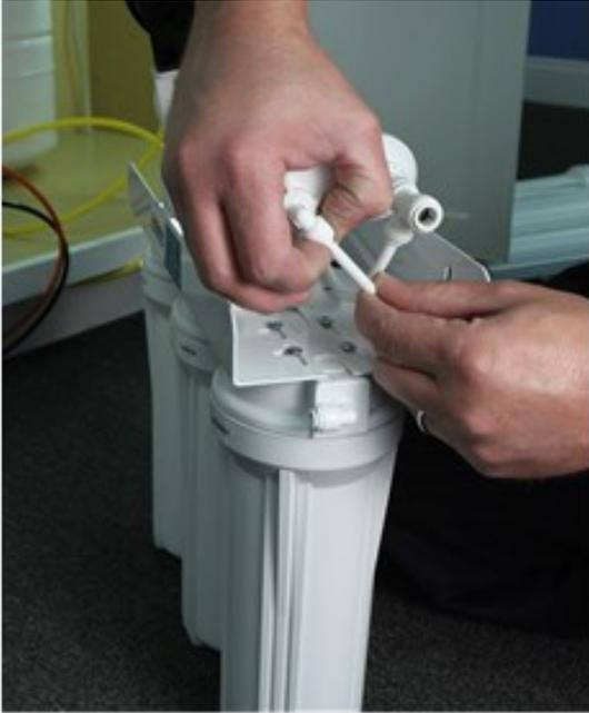
3. Remove the membrane from the protective packaging and install it in the membrane housing. There are two O-rings on end of the middle membrane tube. Lightly lubricate these O-rings with the supplied silicone grease.
