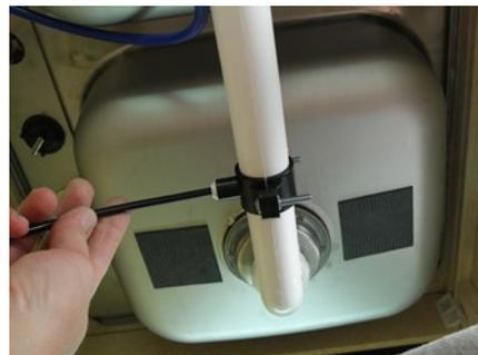
2. Drill 1/4" hole at mark through one side of pipe. **CAREFUL** not to drill through both sides of the pipe.
