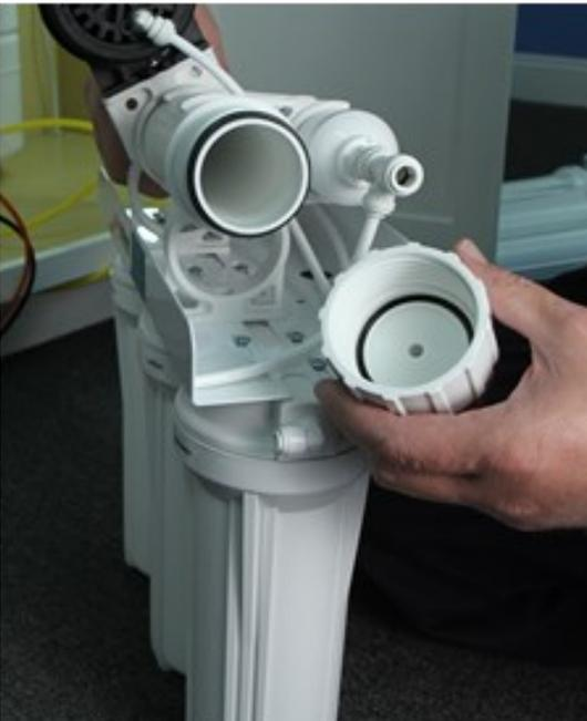
4. **BE SURE** the membrane is fully seated in the housing. If the membrane is fully seated, it will be about 1/8 - 1/4 inset from being flush with the housing.
